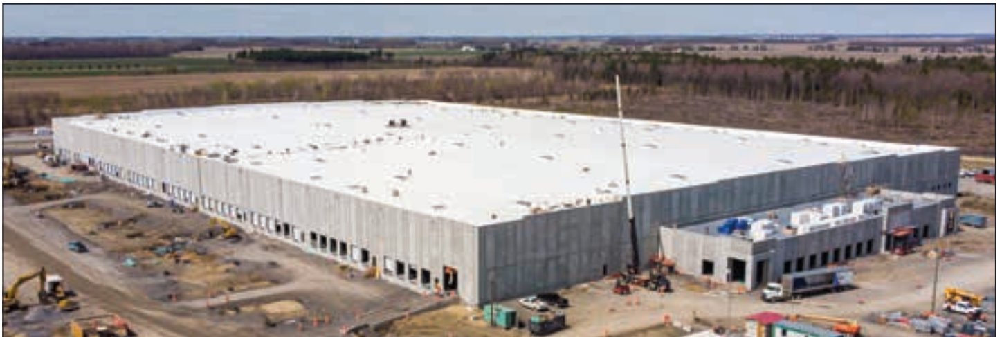
Broccolini: Amazon Distribution Center | Coteau du Lac, Quebec
